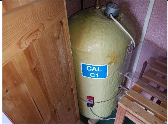
Redundant calorifier
