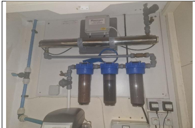
UV PLANT WITH 2 X MICRON FILTERS
