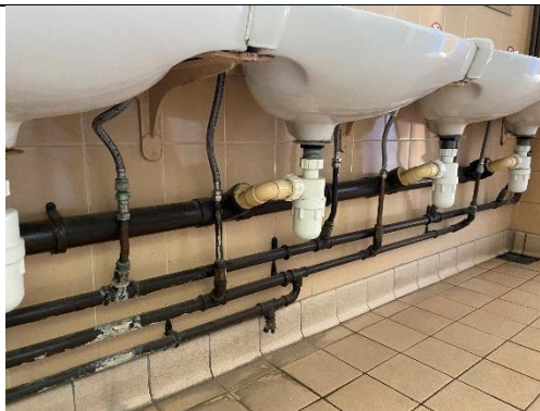
Example of the use of flexible hoses (male toilet basins)
