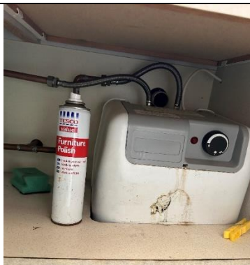
Flexi's on water heater
